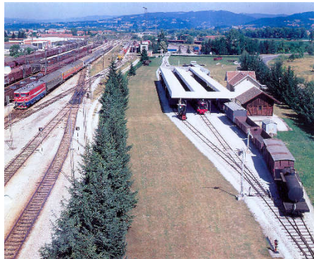
Figure 1: The Department of narrow-gauge railroad in Požega
